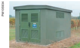
Fig G Example of HV/LV prefabricated substation with 1250 kVA liquid filled transformer, 19 kW of losses before EU regulation change
